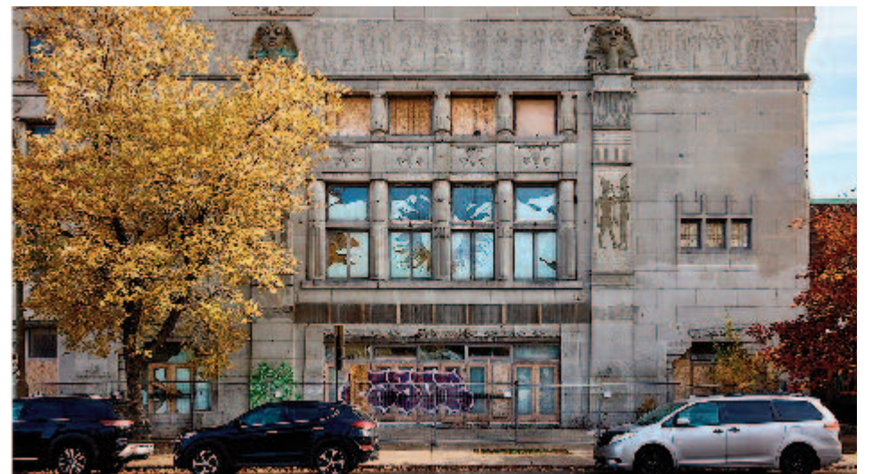
Montreal is preparing to sell the old Empress Theatre in NDG for mixed-use development, following years of efforts to preserve the 1920s Egyptian Revival-style building. Empress Theatre Photo by D. Benjamin Miller
